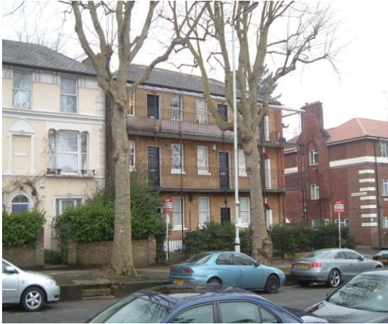
Verandah Cottages, 63 North Hill
